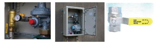
• Turn the valve to the 'off' position. It is off when the lever is at a right angle to the pipe. The gas is on when the lever is parallel to the pipe
